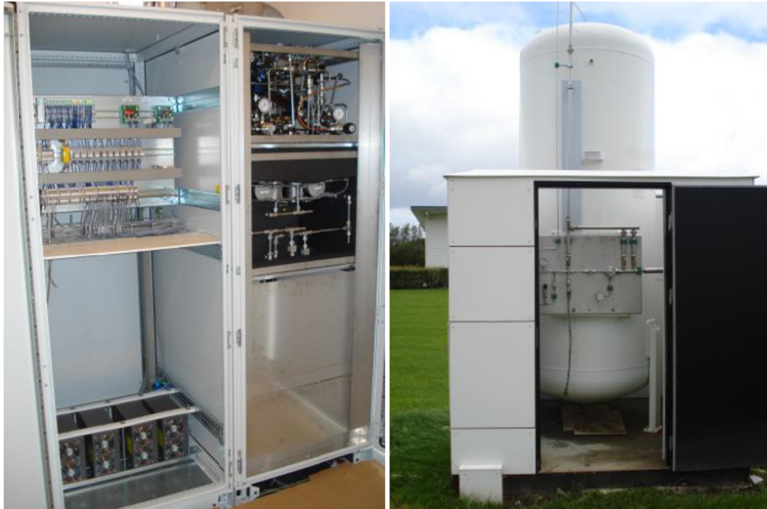
Fig. 27: Left: The electrolyser system used for H2-College. Right: The hydrogen storage tank from H2-College,
