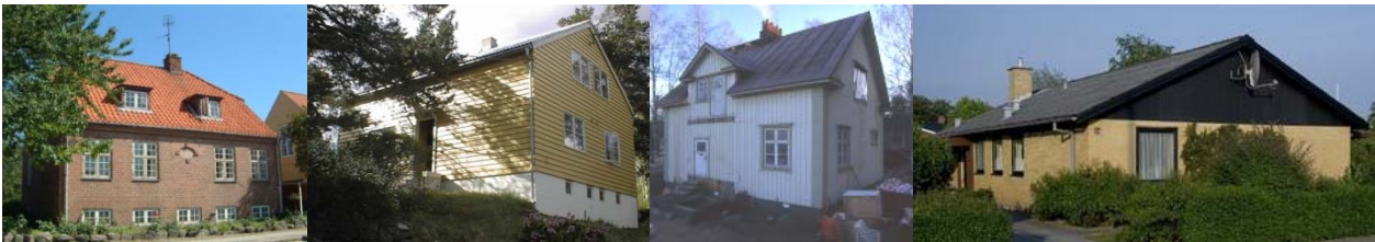
Fig. 2 Typical single-family houses in the Nordic countries. From left to right: Danish house built before 1945, Norwegian house built before 1945, Post-war Finish house, Danish house built in 1960/70's.
