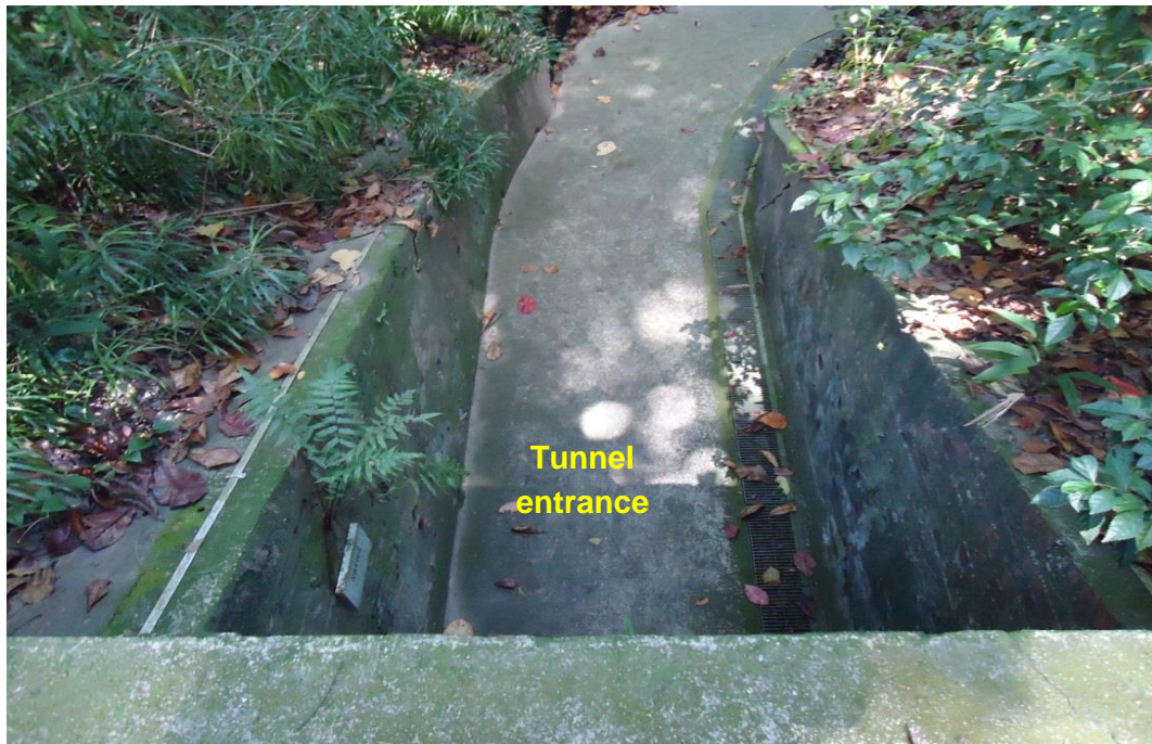
Figure 5-5 Picture of tunnel entrance showing that tunnel is made up of concrete walls
