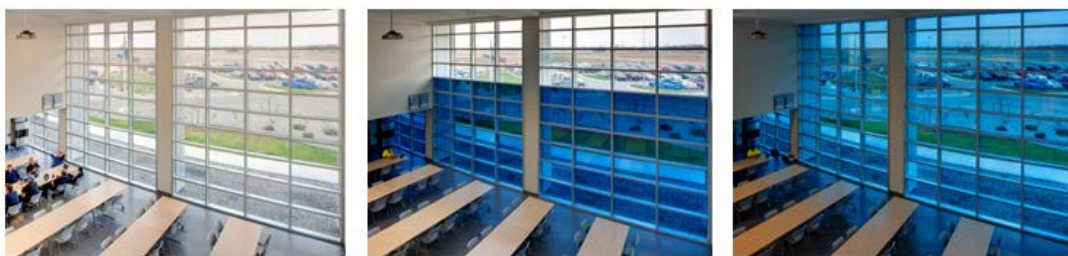
Figure 1-4: Electrochromic windows from Sage Electrochromics at Siemens wind turbine factory in Hutchinson, Kansas. Reprinted from ref 30.
