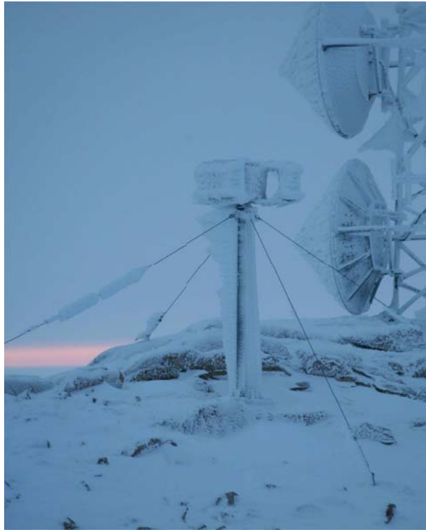
Figure 2.2: A small vertical axis wind turbine located at one of the relay stations in Greenland (photo credit: TELE Greenland).
