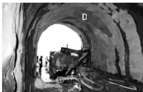
Figure 4 – The area of event: the shotcrete machine and (D, top-right) the area interested by the cementfall.
