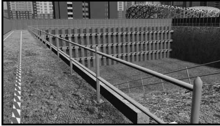
Figure – 4 Excavation border without precaution / with precaution
