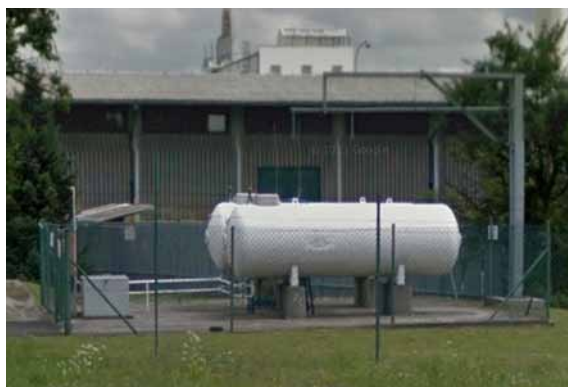
Figure 8 – LPG filling station after installed spraying equipment.
