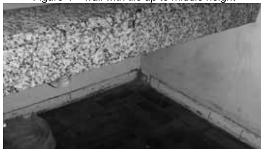
Figure 5 – wall with infiltration and damaged baseboards
