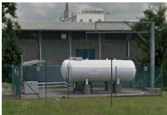
Figure 8 – LPG filling station after installed spraying equipment.
