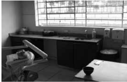
Figure 3 – Windows with no protection against sunlight
