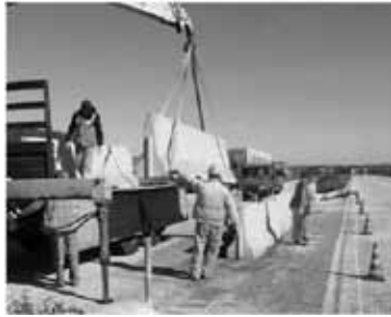
Figure 3 (left) – barrier transfer: traditional procedure; Figure 3 (right) – mechanized “Barrier Zipper” technique.
