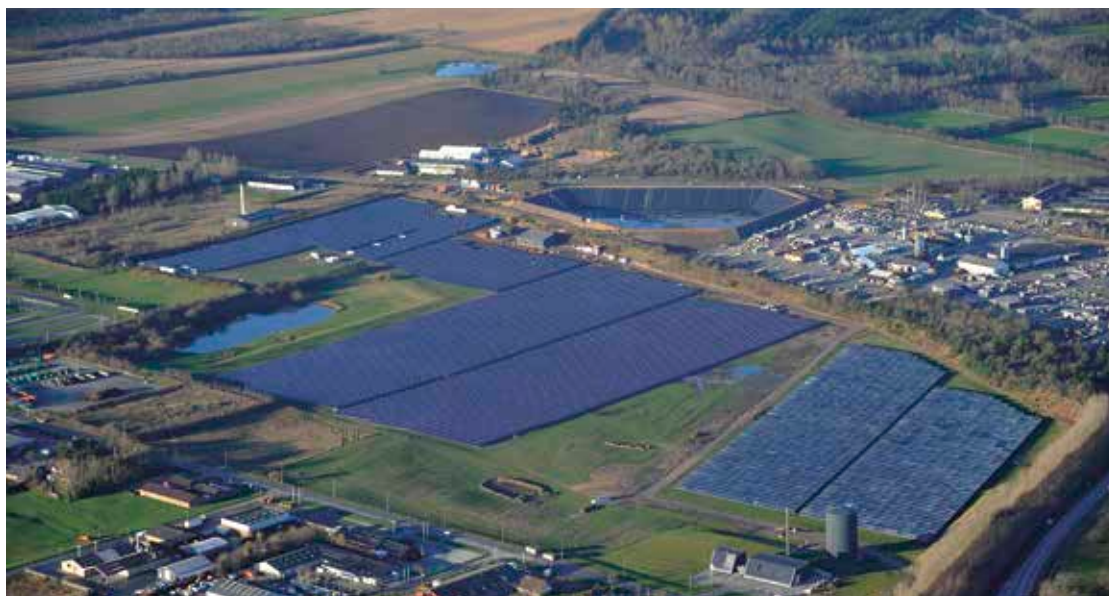
Figure 28 - Vojens solar heating plant with a solar collector area of 70,000 m 2 , the World's largest solar heating system with start of operation in June 2015 [9.8].
