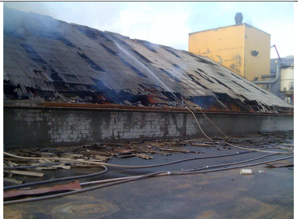
Figure 4 The many light fibre cement roofing panels that remained in place indicate that the explosion overpressure was modest. Note that the wall made of lightweight porous concrete blocks shows no blast damage. Wood dust compartment wall dividers are visible inside building. Photo taken from south. Photo courtesy: Beredskab Vesthimmerland (the local fire and rescue services) photo kindly provided by official of the county Vesthimmerland Kommune.
