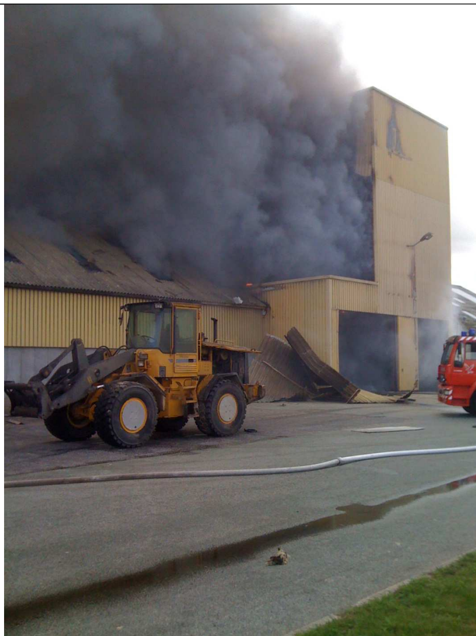
Figure 3 Photo taken one hour after the explosion. The wheel loader is similar to the accident wheel loader, note blown out wall panels. Picture taken from north. Photo courtesy: Beredskab Vesthimmerland (the local fire and rescue services) photo kindly provided by official of the county Vesthimmerland Kommune.
