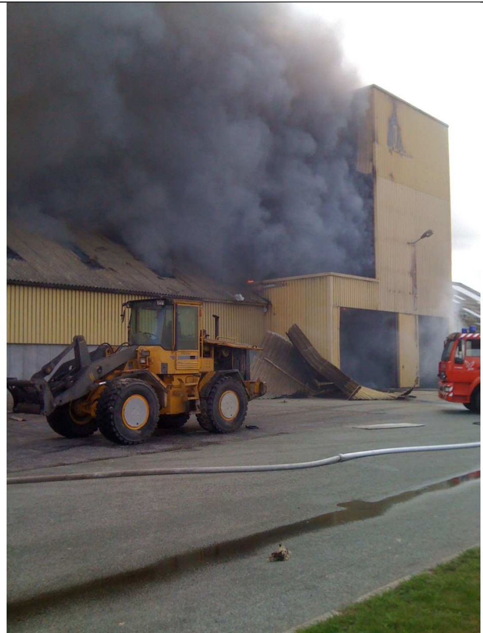
Figure 3 Photo taken one hour after the explosion. The wheel loader is similar to the accident wheel loader, note blown out wall panels. Picture taken from north. Photo courtesy: Beredskab Vesthimmerland (the local fire and rescue services) photo kindly provided by official of the county Vesthimmerland Kommune.
