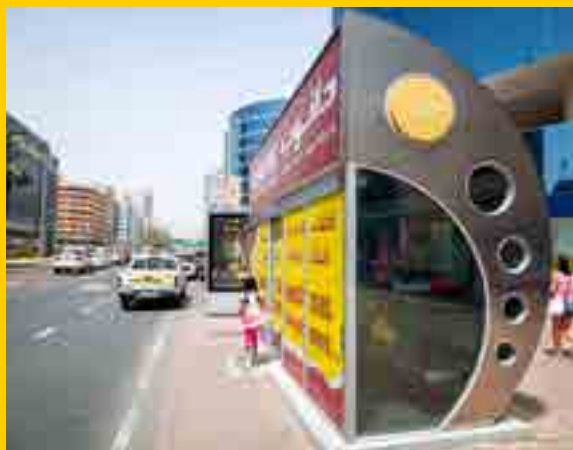
Solar-cooled bus stop in Dubai
