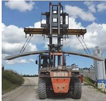
Fig. 1 Four-point transportation of a 13 m Pearl-Chain arch by truck.
