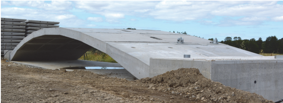
Figure 2: Two adjacent PC-Arches after assembly and lifting.
