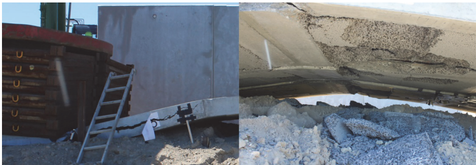
Figure 58: Photographs taken after collapse: longitudinal crack at 3/8 point (left) and crushed LAC at 5/8 point (right).
