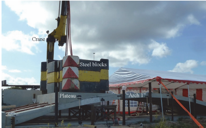
Figure 11: Test 1. Six steel blocks, each weighing 10 tonnes, were set on the plateaus on “arch 1” (near side in photograph) and “arch 2”.
