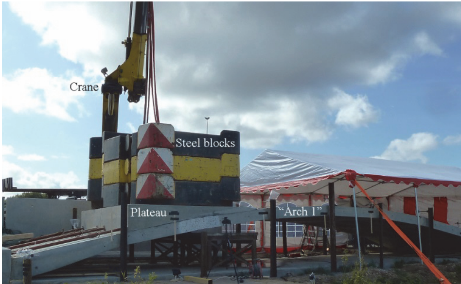
Figure 49: Test 1. Six steel blocks, each weighing 10 tonnes, were set on the plateaus on "arch 1" (near side in photograph) and "arch 2".
