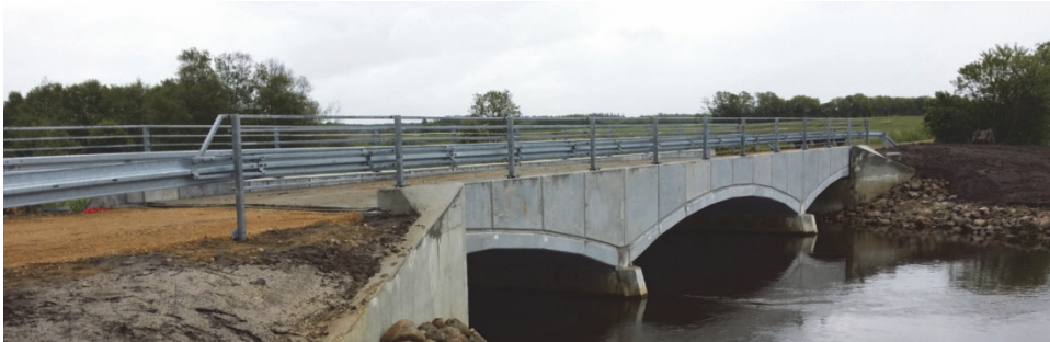
Figure 60: The finished Vorgod Creek PC-Bridge. Courtesy of Abeo A/S.
