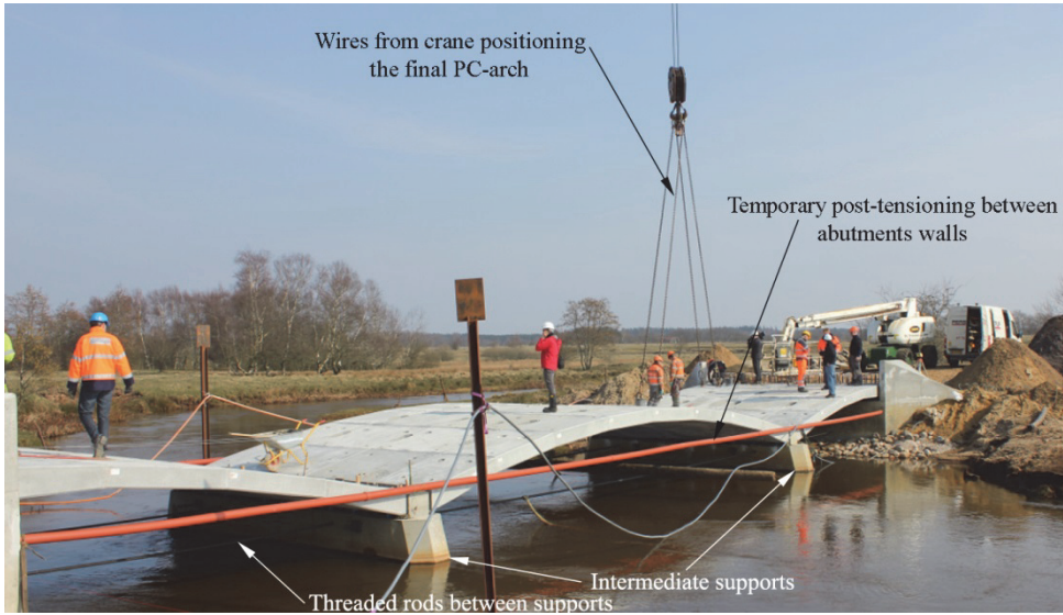
Figure 65: Vorgod Creek Bridge after erection of the 12 PC-arches.
