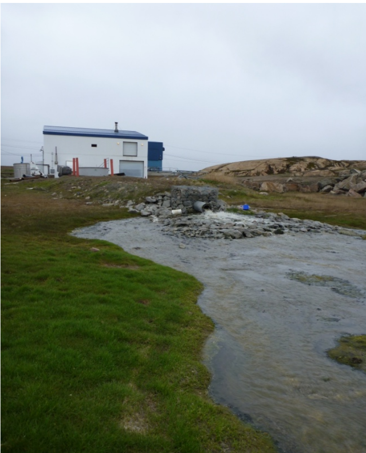
Figure 1. Mechanical wastewater treatment system in Iqaluit, Nunavut
