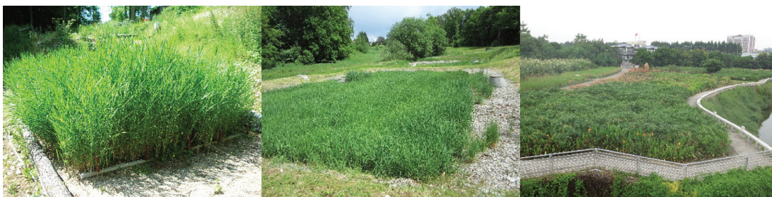
Figure 1. Wetland systems are commonly used for secondary treatment (left: vertical flow wetland in Austria; middle: horizontal flow wetland in the Czech Republic) and for tertiary treatment of domestic wastewater (right: tertiary treatment wetland near Shanghai, China). (Pictures: Günter Langergraber.)
