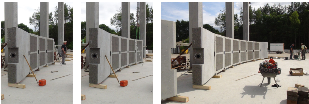
(a) One abutment element and three SL-Decks. (b) One abutment element and four SL-Decks. (c) Two abutment elements and six SL-Decks.
