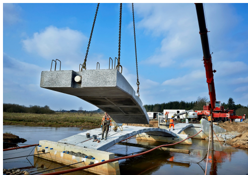
(a) Emplacement of Pearl-Chain arch.
