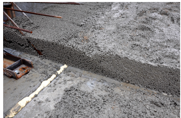
Fig. 7. Difference in consistency in PCPC placed in third layer of filling material on Pearl-Chain Bridge over Vorgod Stream. PCPC close to the bridge center (right hand side of photo) is considerably wetter than PCPC close to the bridge edge (left hand side of photo).
