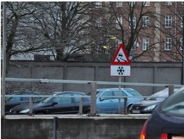
(a) Bispebuen bridge, Copenhagen.
