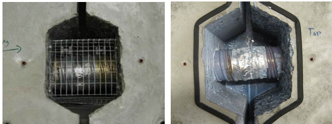
(c) Shrinkage crack reinforcement with a mesh size of 1 cm × 2 cm installed around the ducts. (d) Surface treatment with water and primer.
