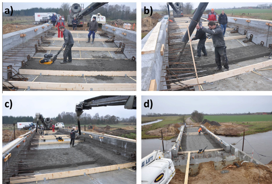
Fig. 6. Filling of pervious concrete on Pearl-Chain Bridge over Vorgod Stream. a: compaction of first layer; b: casting of second layer; c: casting of third layer; d: finishing of fourth layer.
