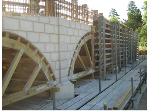
(b) This typical scaffolding used to construct an arch structure is expensive and requires many labor hours to complete. Photo: http://www.idh-design.co.uk/news/rebuilding-of-the-five-arch-bridge .
