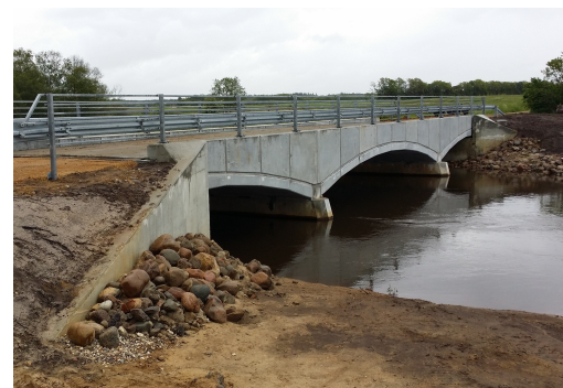
(b) Finalized Pearl-Chain Bridge crossing Vorgod Stream.
