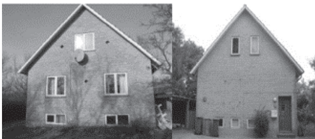
(a) Back facade (b) Front facade
