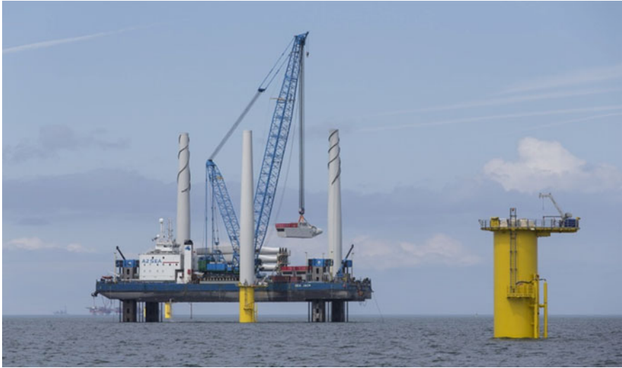
Fig. 19.1 A2SEAs SEA JACK during the construction of the Gwynt y Mor wind farm. Image Source: A2SEA (2016)
