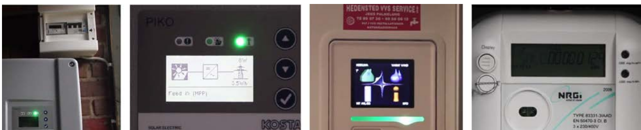
Figure 1. Examples of the displays installed in the 20 households. Left: The first and second photos resemble the inverter. The third photo shows the HP-display. The fourth photo shows the smart metre display (courtesy of Insero).
