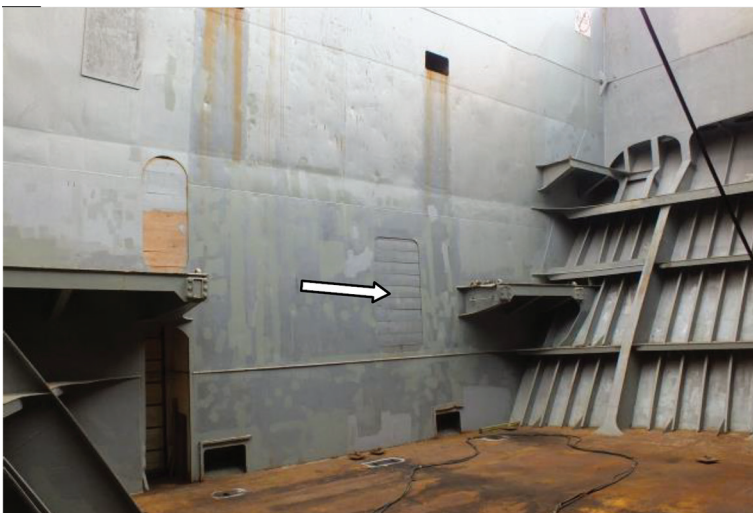
Figure 3. An opening in the front cargo hold allowed easy access to the lashing equipment room. When carrying bulk cargo, the opening was closed with planks of wood inserted into guide bars (CORINA). Source: [16].
