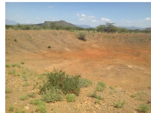
Photo 3: Poor design and siting of water pans limits the technology ability to retain water throughout the dry season observed in Isiolo
