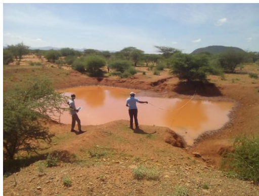
Photo 3: Siltation remain the key challenge affecting the functionality and durability of water pans
