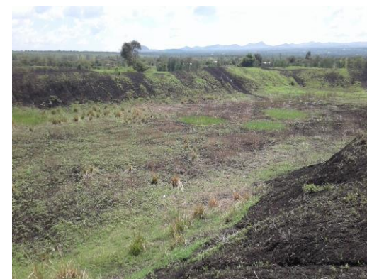
Photo 3: Poor design and siting of water pans limits the technology ability to retain water throughout the dry season observed in Isiolo
