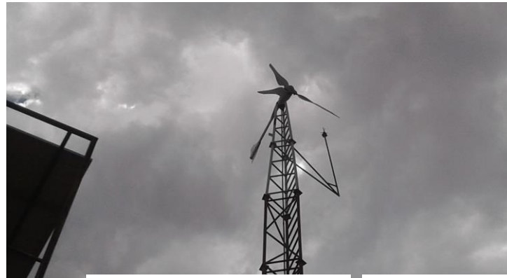
Photo 5: Hybrid system solar and small wind turbine in Baringo County. The system is not functional since the submersible pump has corroded due to high water salinity
