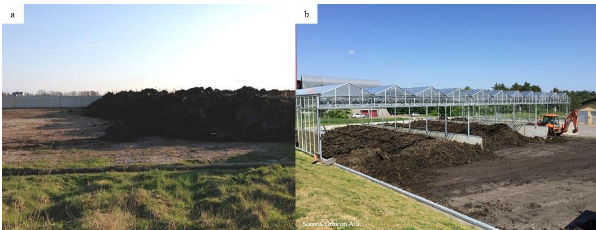
Figure 6: a) Sludge residue piled on the stockpile area at Himmermark WWTP in 2014. b) Sludge residue piled at the stockpile area at Helsingør WWTP in 2016. The area is covered by a greenhouse roof, and greenhouse walls on two sides.
