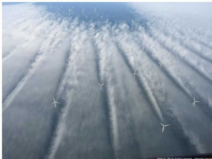
Figure 1: Photograph of the Horns Rev 2 offshore wind farm on 25 January 2016 at 12:45 UTC seen from SSW direction. Photo by Bel Air Aviation Denmark, Helicopter Services. Source: Hasager et al. 2017 Energies doi:10.3390/en10030317
