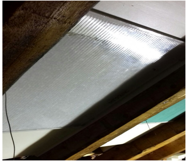
Fig.2 Installation of a PCM filled panel
