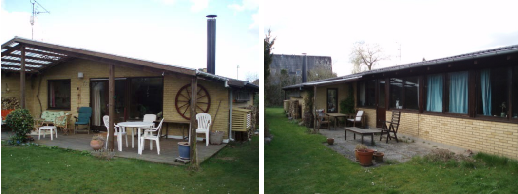
Figure 2 – The house before the renovation as seen from west and southeast.
