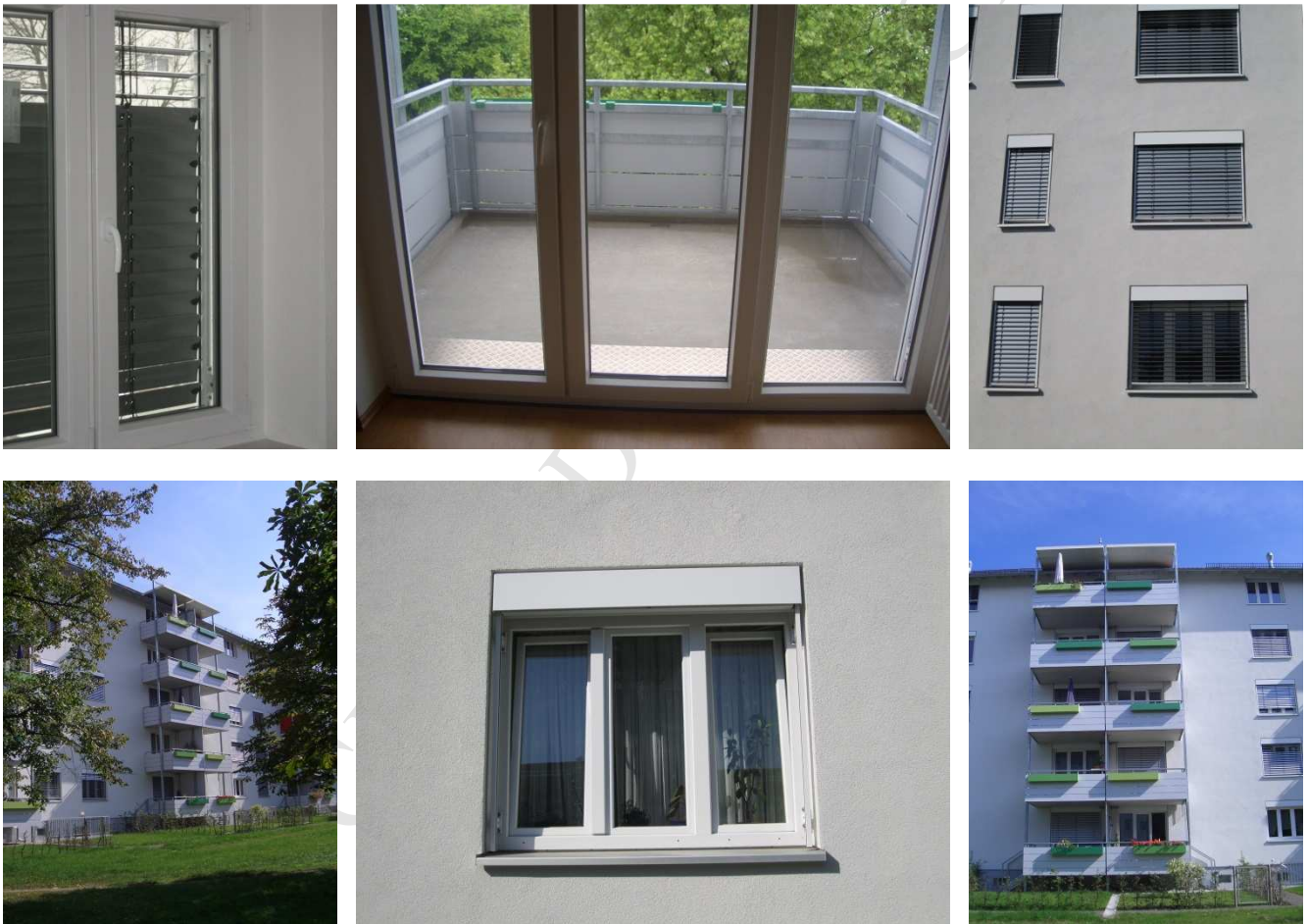
17 18 19 Figure 4. Pictures of the windows and of the façade after retrofit.
