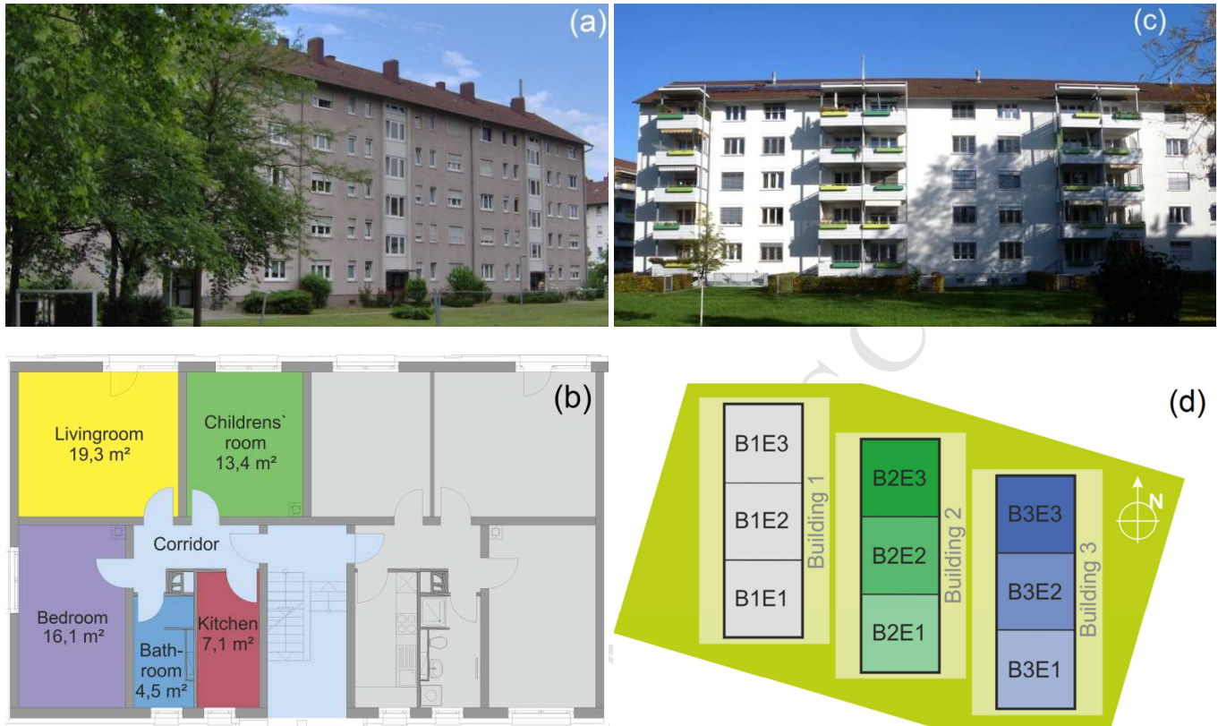
6 7 8 Figure 3. One building façade before retrofit (a). One back façade after the retrofit (c). Floor space of the apartments, for one 9 entrance with south-gable (b). Relative position and orientation of the buildings (d).
