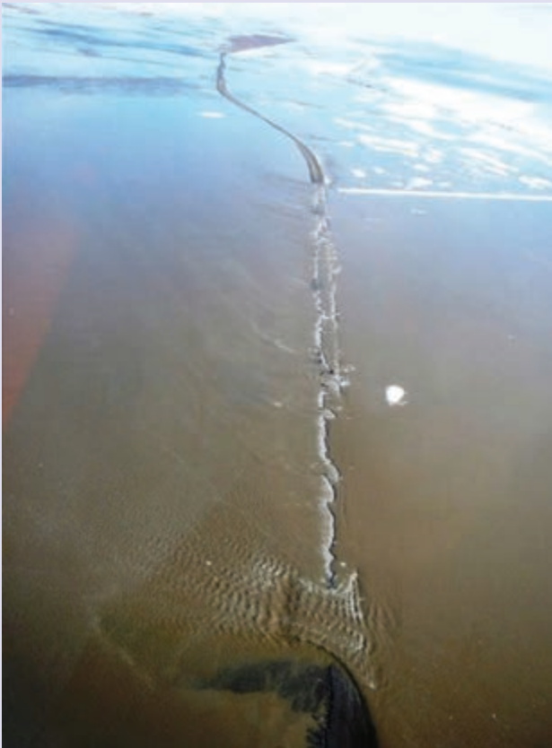
Figure 4.28 Area of major washout during the height of the flood on 19 May 2015 (photo: KTUU News).
