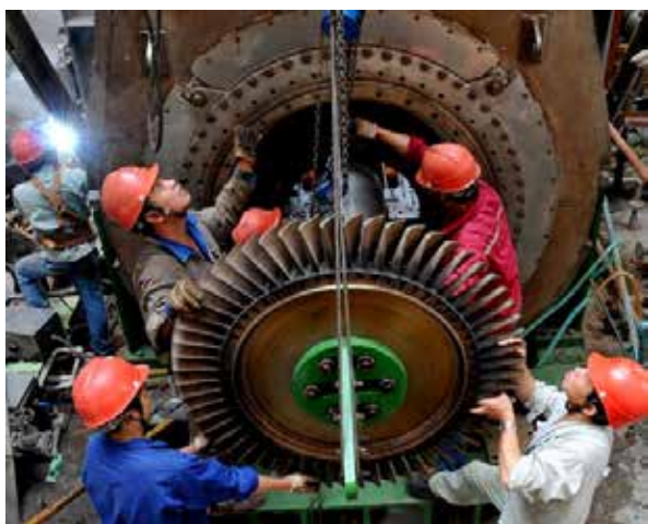
FIGURE 4. Energy Conservation Retrofit in a Power Plant
