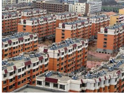
(c). Solar water heaters
