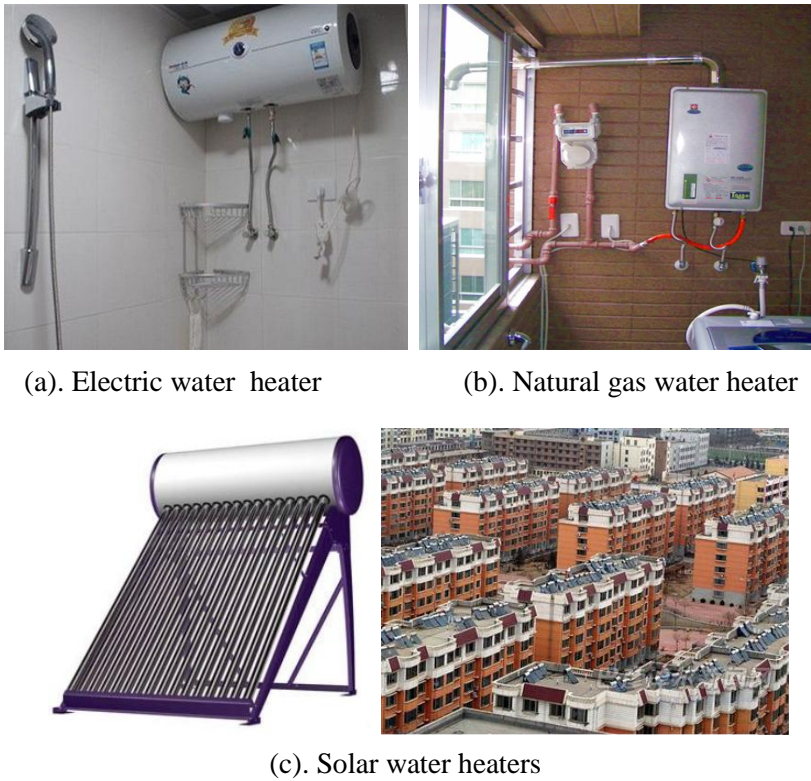
Figure 2. Individual water heater installations in Chinese households
