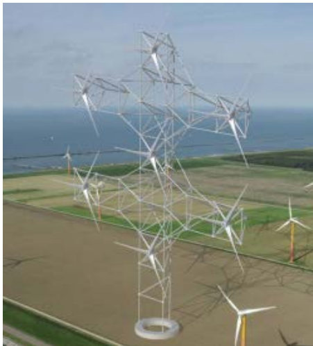
Figure 2.3. 3-Rotor turbine concept by Hermann Honnef, 1930 [9]
