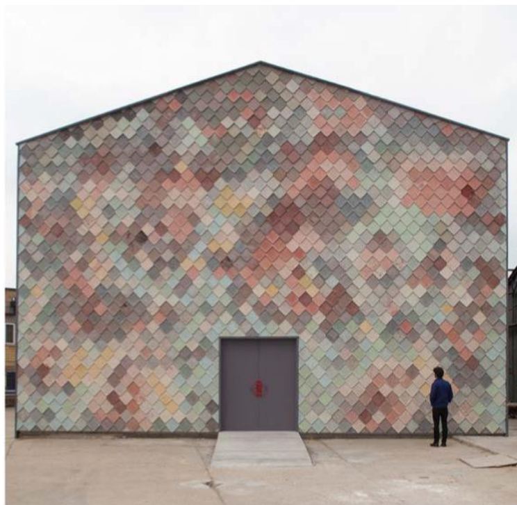
Fig. 7. Yardhouse, 2014 by Assemble. The facade is made from concrete tiles. The colourful tiles is hand made on site. Photo:ASSEMBLE
