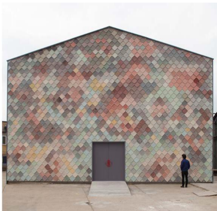
Fig. 7. Yardhouse, 2014 by Assemble. The facade is made from concrete tiles. The colourful tiles is hand made on site. Photo:ASSEMBLE
