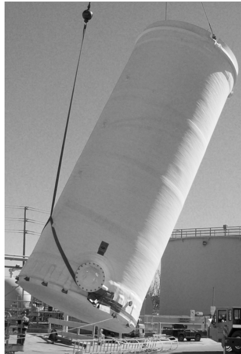
Figure 2.11: Example of a FRP tank made of Derakane vinyl ester [70]. Courtesy of Ashland Inc. and Owens Corning
