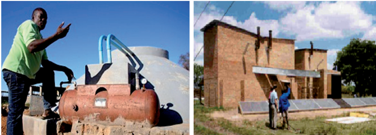
Figure 11.5 Use of biogas digester at Victory Farm (Beatrice) and solar application in tobacco barns
