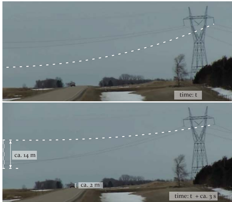
Figure 1.2: Documented galloping event: 345 kV transmission line system with galloping conductor lines in a 1-loop mode (South Dakota, USA), [11].
