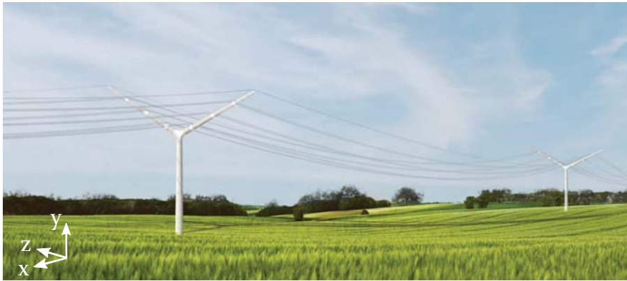
Figure 1.1: Composite power pylon with directly attached overhead transmission line bundles, [6].
