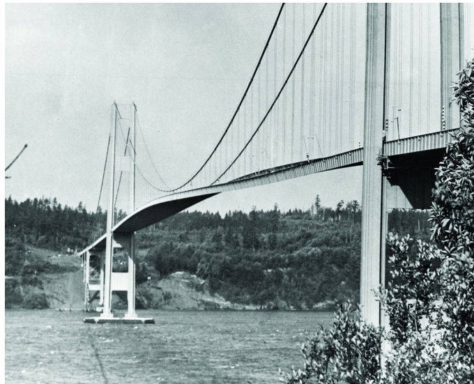
Figure 1: Large amplitude torsional oscillations of the first Tacoma Narrows Bridge in 1940.
