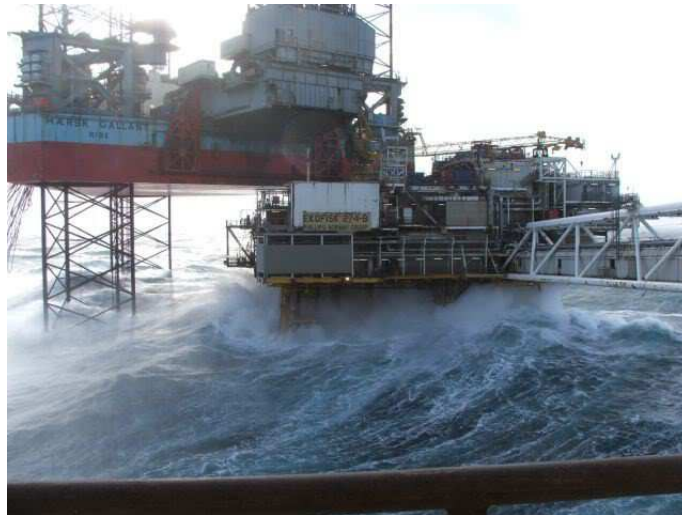
Figure 1.1. Wave-in-deck event at Ekofisk. 1
