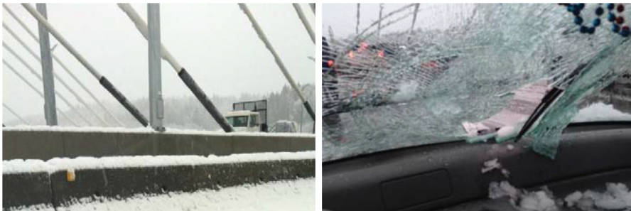
Figure 2.14 – Ice formation on the cable sections of the Port Mann Bridge in Vancouver, British Columbia (a); damage to passing car (b). (Pictures from http://www.vancouver.sun.com ).
