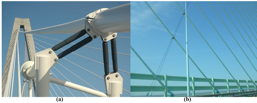
Figure 2.12 – Examples of (a) dampers between the cable and the bridge girder (From http://ravenelbridge.net/freyssinet.php ), and (b) cross-ties between cables (From https://failures.wikispaces.com/Cable+Bridge+Failures+Overview ).
