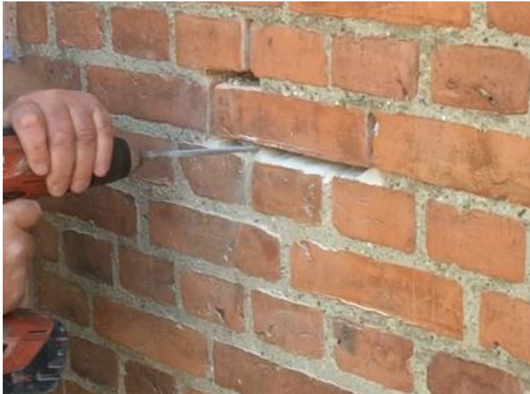
Figure 1: Removing the brick from the wall at Dr. Sellsvej 39, Building 9
