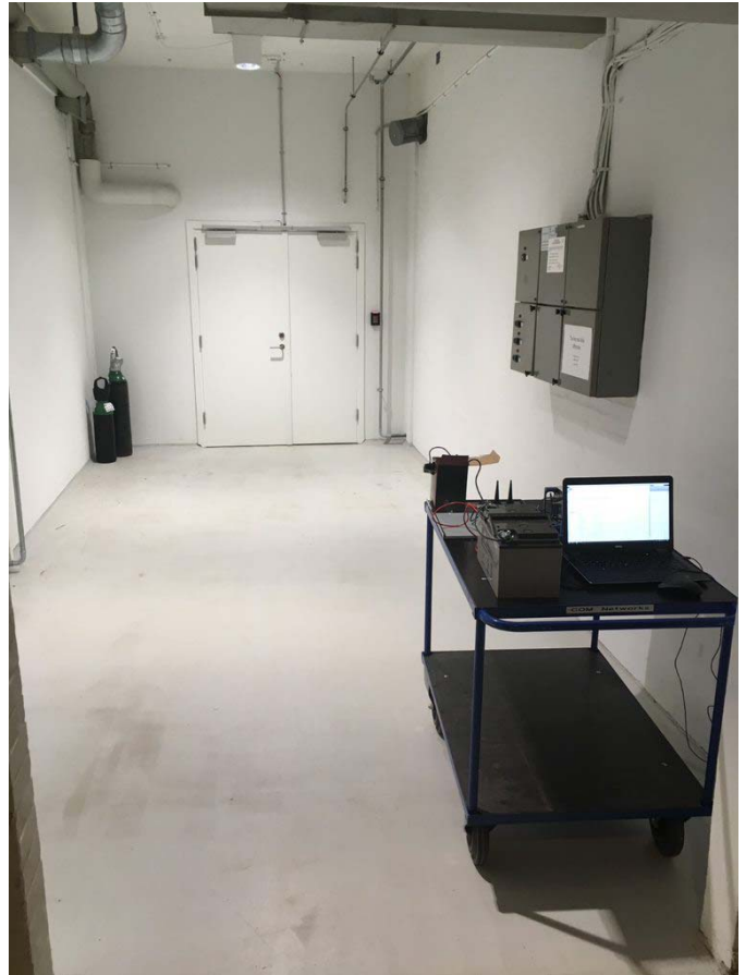
Fig. 5. Measurements in the basement of building 340
