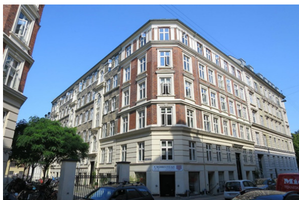
Fig. 1. Case study building.
