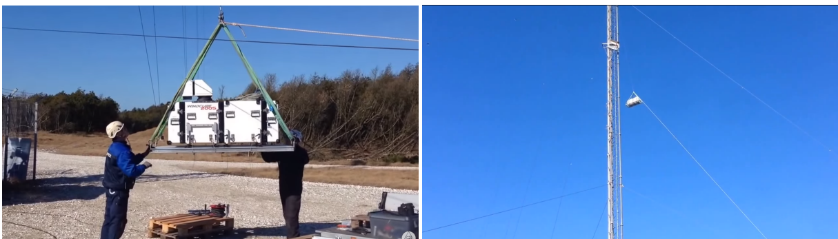
Figure 2. Photos of the lidar platform during the lifting procedure
