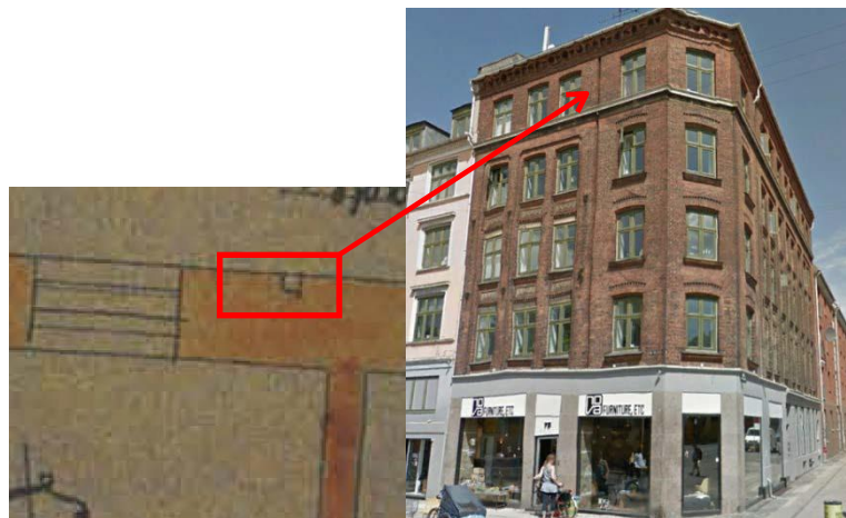
Figure 11: Indent in wall by sensor 6
