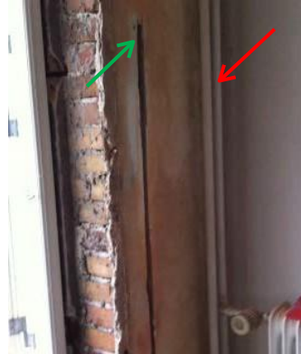
Figure 15: Hot water pipes (red arrow) in the vicinity of sensor 6 location (green arrow)
