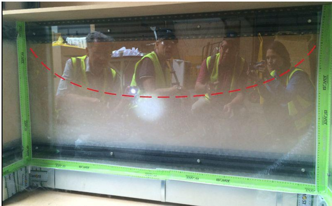
Figure 48: Movement of air beneath window visualized with smoke test
