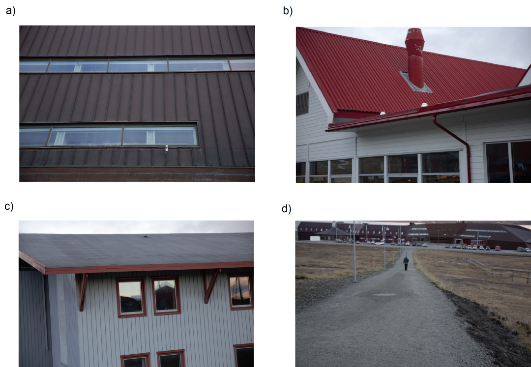
Figure 2. Examples for roof and road types considered in Lu et al. [54] for Longyearbyen (object ID in ()): (a) pitched metal roof, dark paint (#1); (b) pitched metal roof, red paint (#5); (c) pitched with roofing felt (#15); and (d) gravel footpath (#21).
