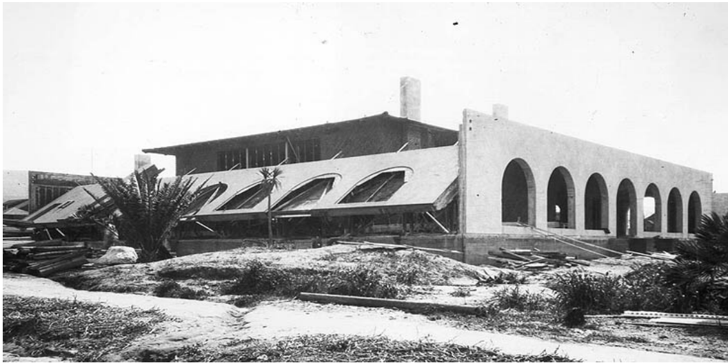
Figure 1.1 Tilt-slab concrete construction for La Jolla Woman's Club built between years 1912 to 1914 (Schaffer, 1998).
