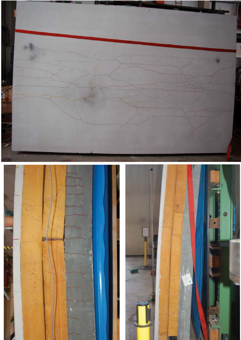
Figure 7.17. Typical failure modes of the panel #02 - test setup 2.
