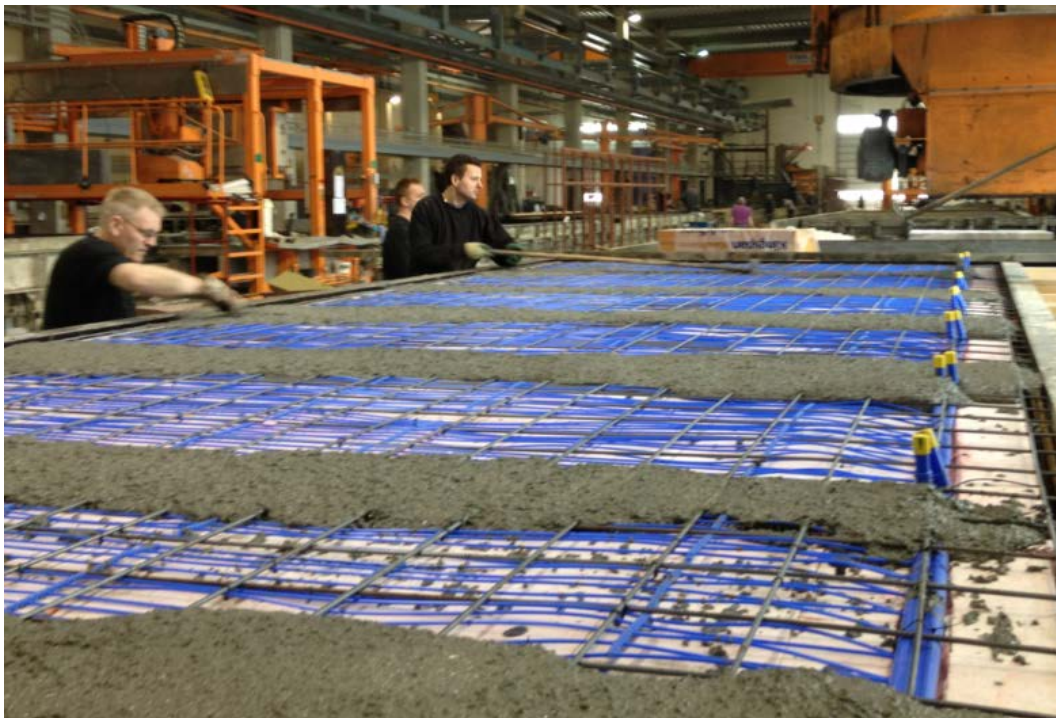
Figure 15: Casting of CPTs in the HPC wall element
