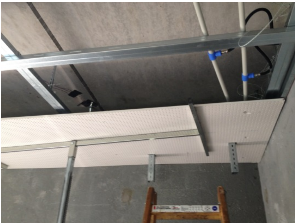
Figure 23: Installation of suspended ceiling
