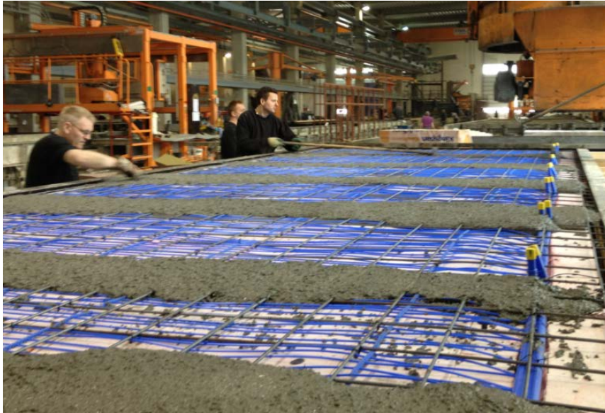
Figure 3: Casting of radiant cooling made of capillary mats
