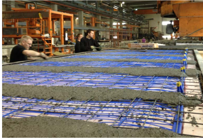
Figure 5: Capillary mats casted into the layer of concrete
