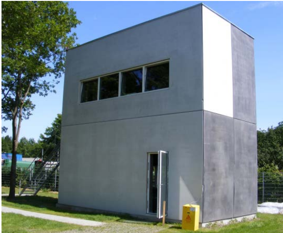
Figure 10: Test House after its construction
