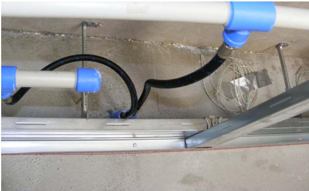
Figure 17: Connection of capillary mats with manifold pipes
