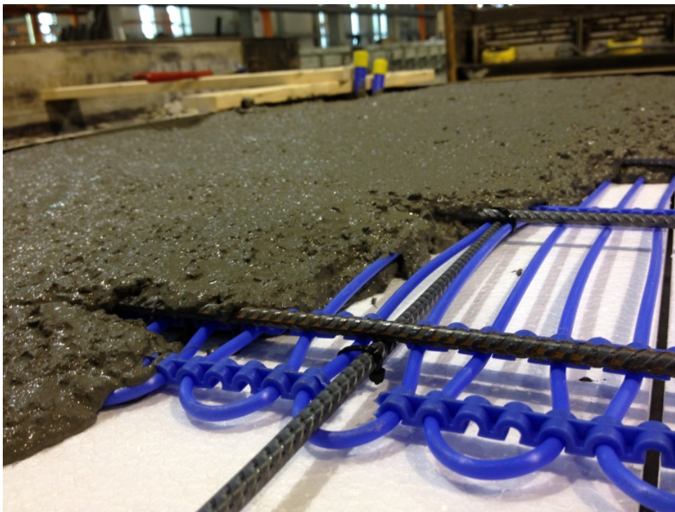
Figure 18: Detail of steel reinforcement in concrete layer
