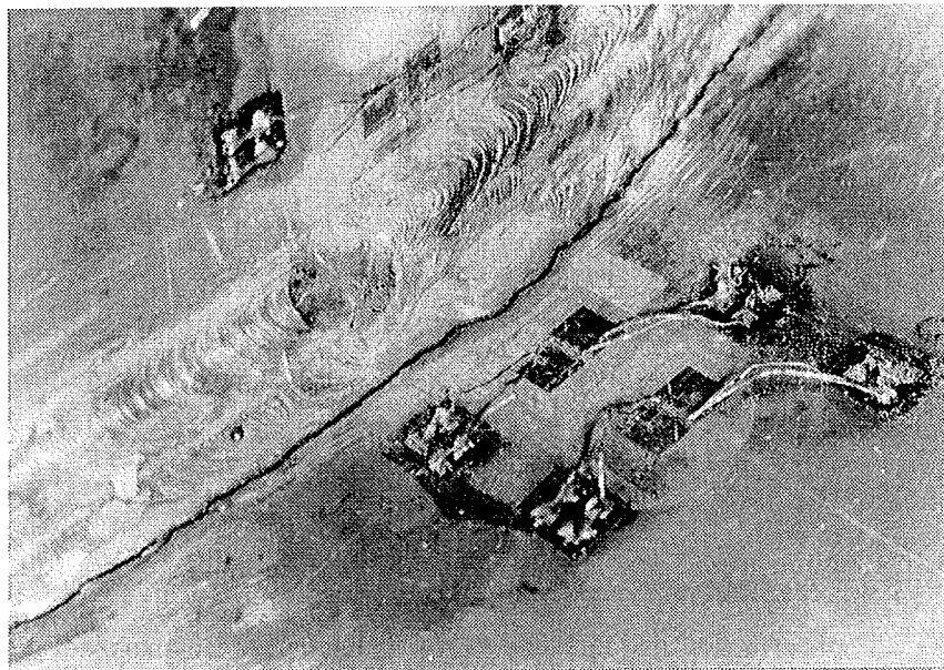
Fig. 4.11 Fatigue crack in chord at edge of weld. Test No. W1.
