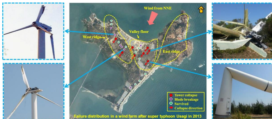
Figure 4. A wind farm located on a coastal island is impacted by a typhoon in 2013 [5]. In total, 35 out of 75 22.9-meter long blades are totally fractured in the wind farm. The fracture location is from 6 to 11 m from the blade root. The estimated wind speed during the typhoon is higher than the design survival wind speed of the turbine.
