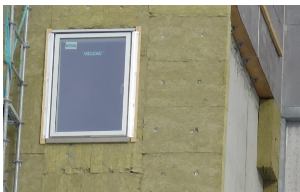
Fig. 4. Building with focus on non-organic materials; outer walls of in-situ cast concrete with mineral wool on the outside. Later a ventilated cladding was installed but no wind barrier.
