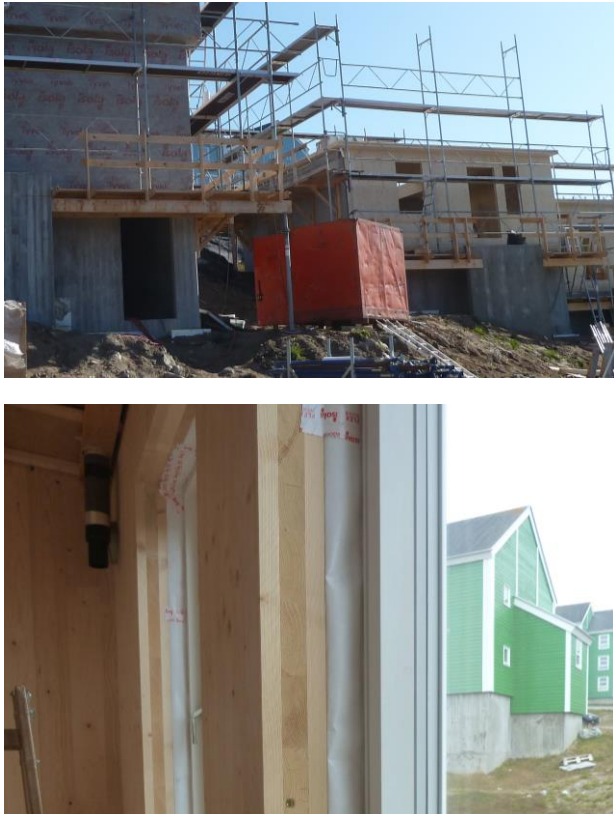
Fig. 6. Two storey double family houses built with CLT elements. The upper photo shows different stages of the process, to the right the raw CLT elements, to the left a diffusion open foil covers the CLT elements before the insulation is mounted. Below is a photo of the inside of the house before the lining is installed.
