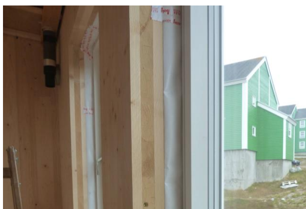
Fig. 6. Two storey double family houses built with CLT elements. The upper photo shows different stages of the process, to the right the raw CLT elements, to the left a diffusion open foil covers the CLT elements before the insulation is mounted. Below is a photo of the inside of the house before the lining is installed.
