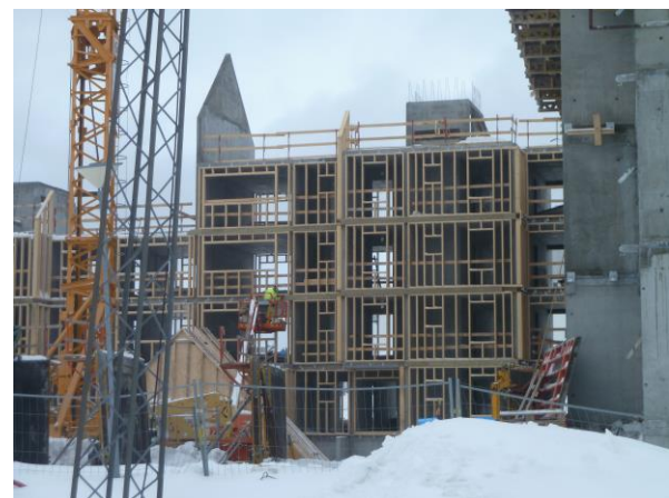
Fig. 2. Example where the traditional building method is used. Gables and interior walls of in-situ cast concrete, façade with timber frame
