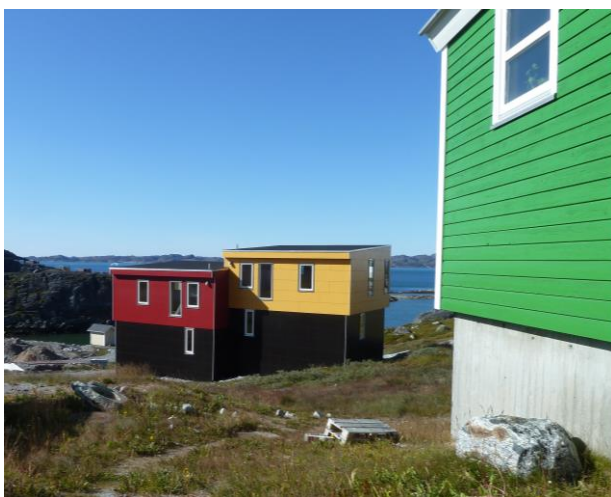
Fig. 8. To limit the need for repainting, alternatives to the traditional colourful cladding (in the front) have become popular; here coloured compressed mineral wool boards cladding for double family houses made of CLT elements, same projects as in Figure 6.
