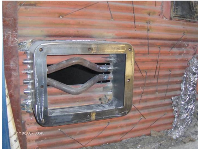
Figure 6 Measurement port welded into the side wall before packing and isolating.
