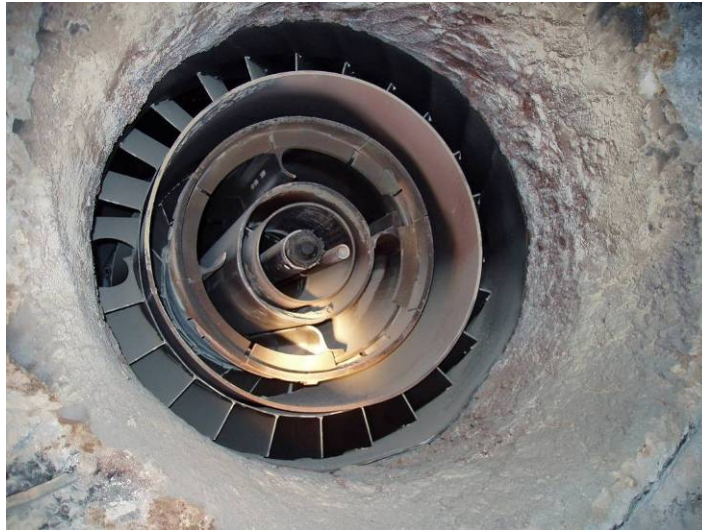
Figure 2 . The Mitsui-Babcock Low-NOx burner in standard configuration.
