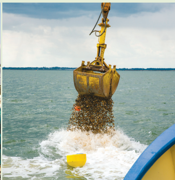
Figure 2.14: Deployment of gravel cultch by Essex Native Oyster Restoration Initiative, UK. Photo: ENORI/ZSL.
