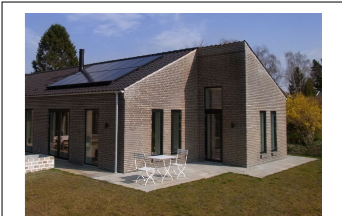
Figure 4-47 A typical new Danish low-energy house. The house is more complicated to operate than an older house due to the larger number of technical installation.
