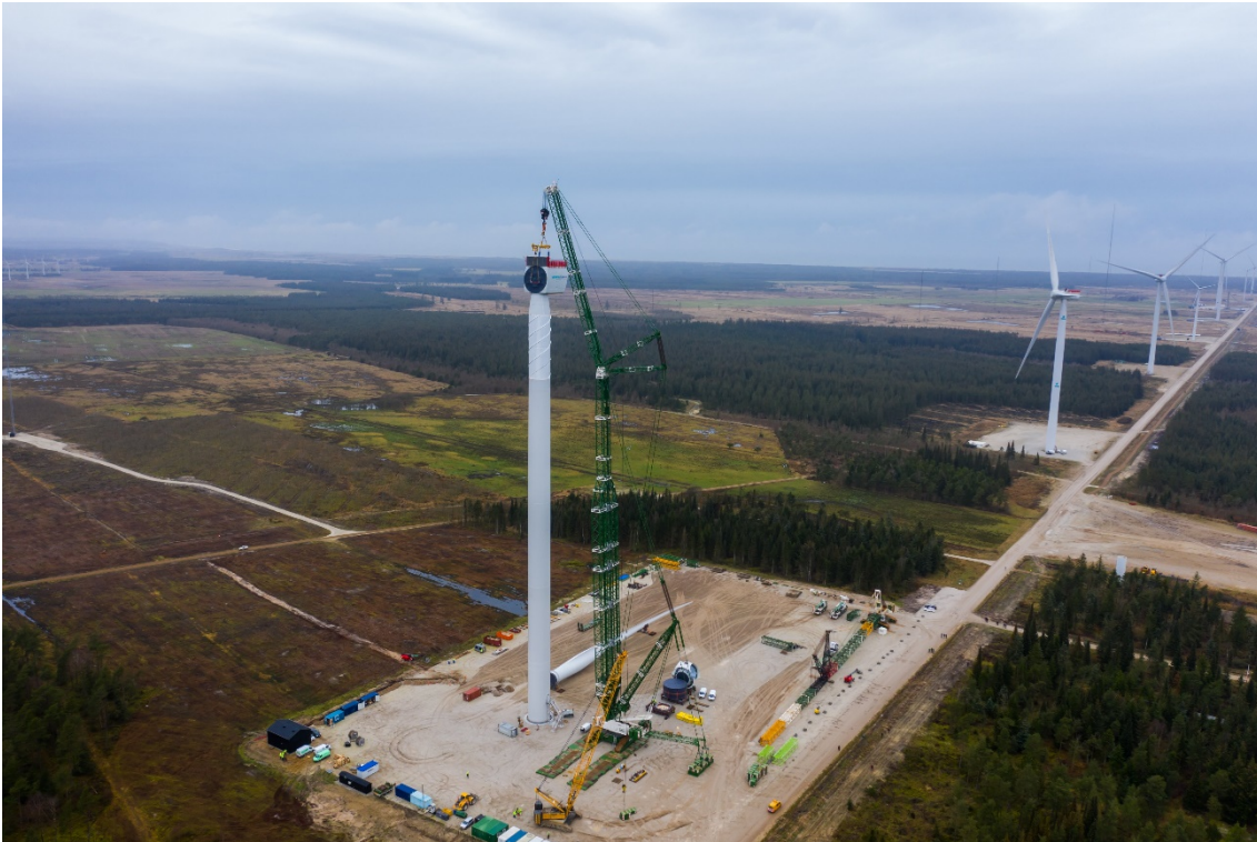
Figure 8. Assembly of Siemens Gamesa 11 MW wind turbine. Photo: Siemens Gamesa
