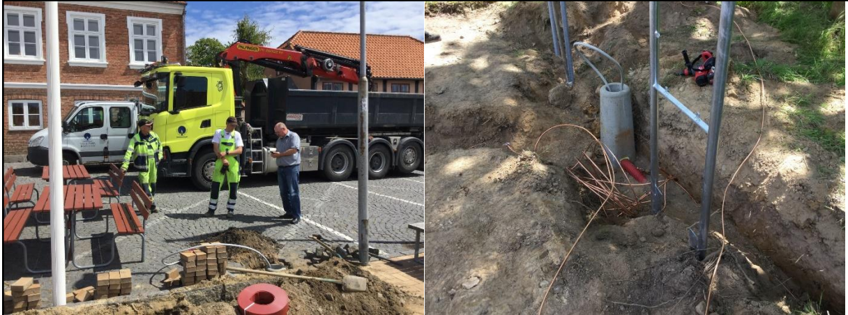
Figure 5. Infrastructure and electric grounding works.
